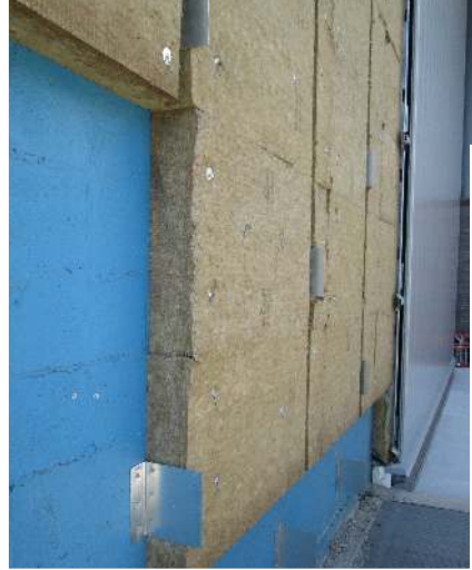
Top & Bottom Right: Completed Reskinning Bottom Left: Conditions Prior to Reskinning Bottom Center: Application of Rockwool Insulation
