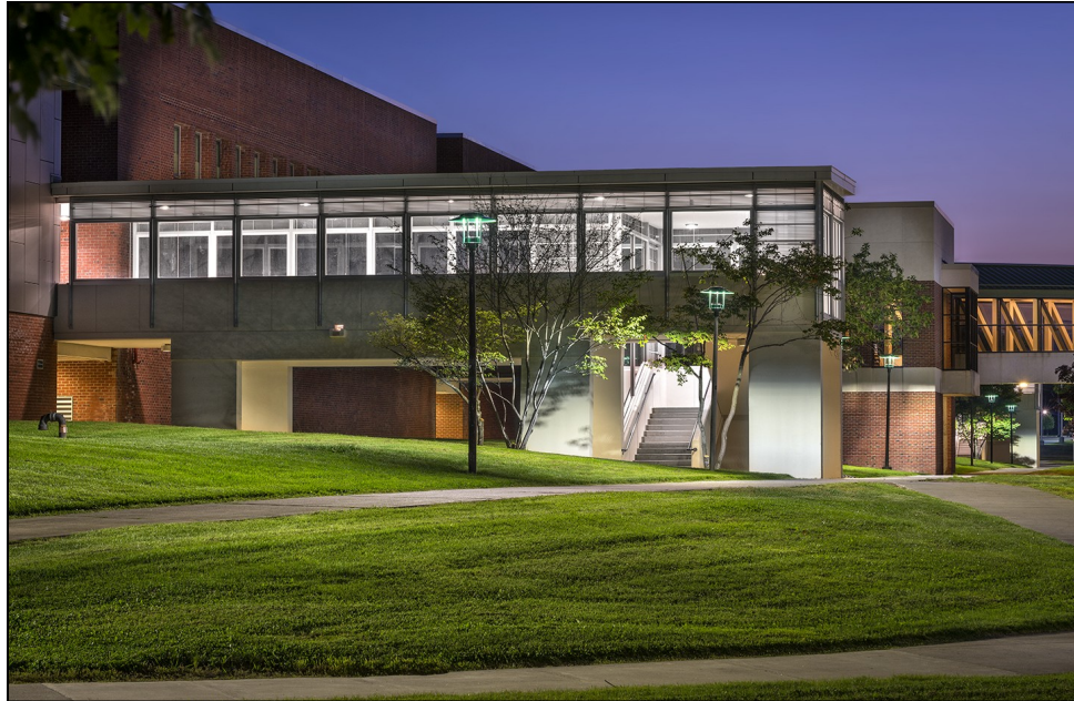
SUNY College at Brockport Entry Walkway at Dusk - Brockport, New York
