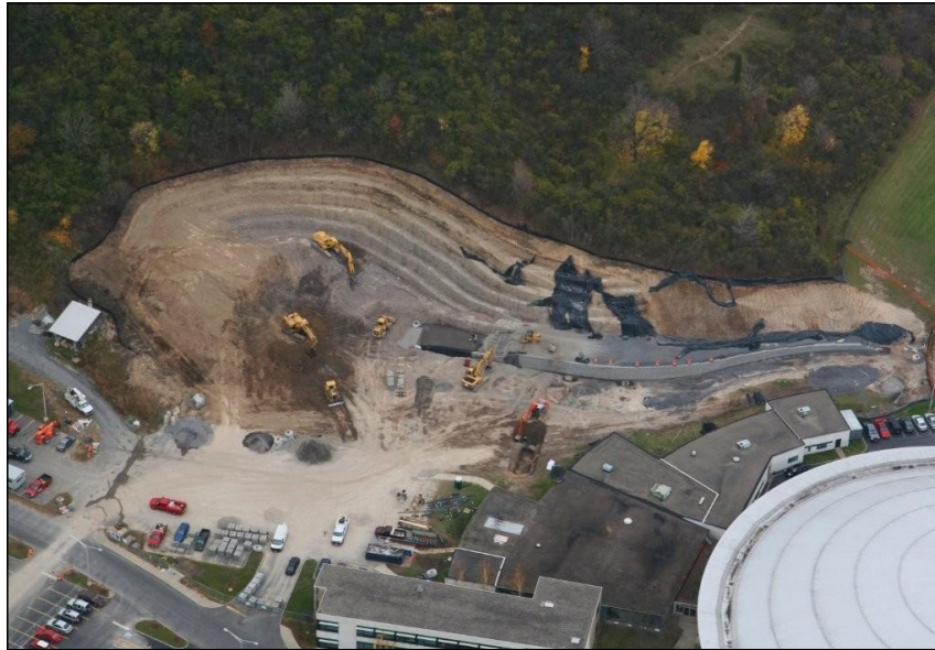
Carmelo K. Anthony Basketball Practice Facility Site Work Aerial View
