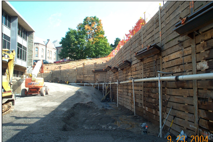
Case Library Site Work at Colgate University
