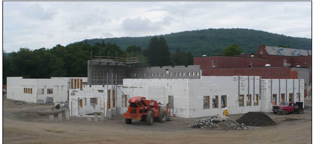
Worcester Central School District Insulated Concrete Form Construction
