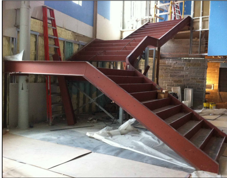
Articulated steel-framed stair at the Sadler Dining Hall expansion
